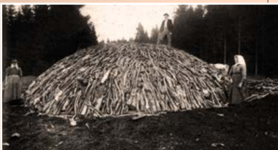
Charcoal oven prior to being covered by peat etc. From Schwarzwald in Germany around 1900
