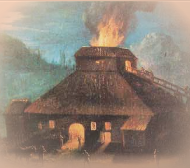
Blast furnace building at Bærums Verk around 1800. Extract of a painting by C.A. Lorentzen
